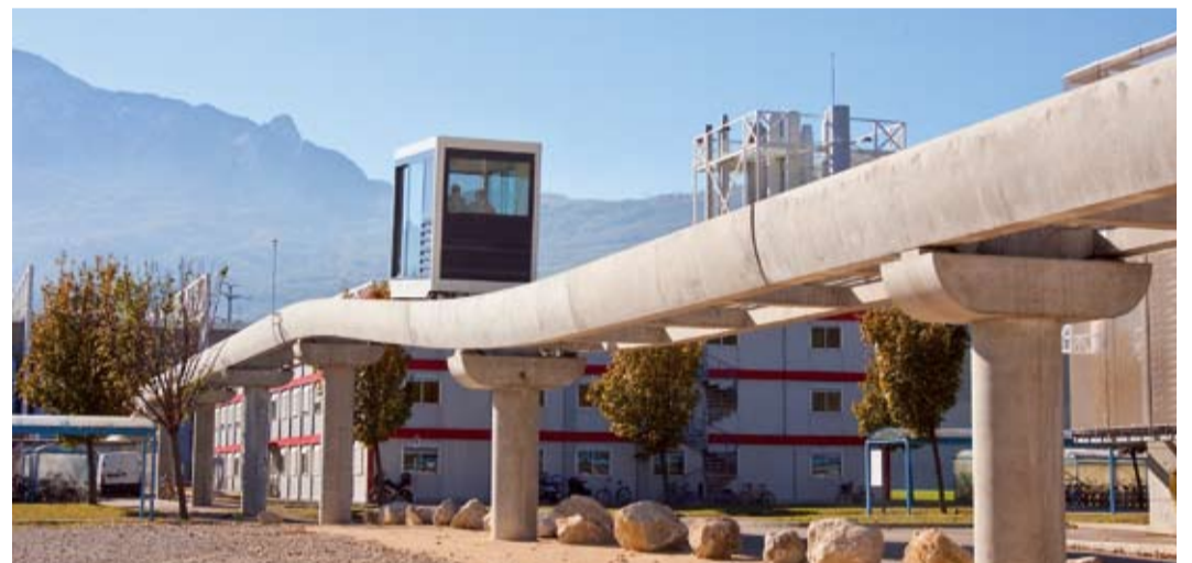
▲ THE "CLEAN-CLEAN" CABIN IN ACTION, ALONG THE 250 M LONG CONCRETE RAIL
