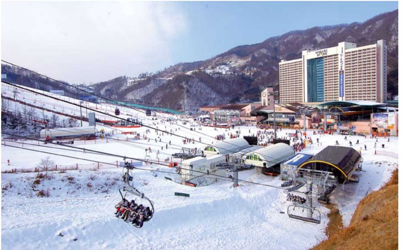
▲ OVERVIEW OF THE STATION
